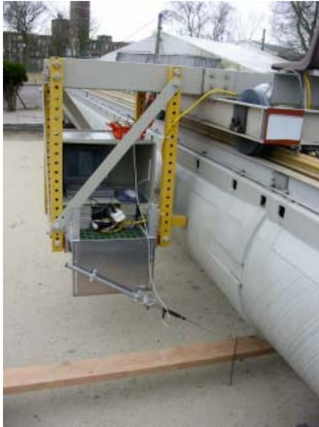
Figure B.5: Picture of the test installation.
