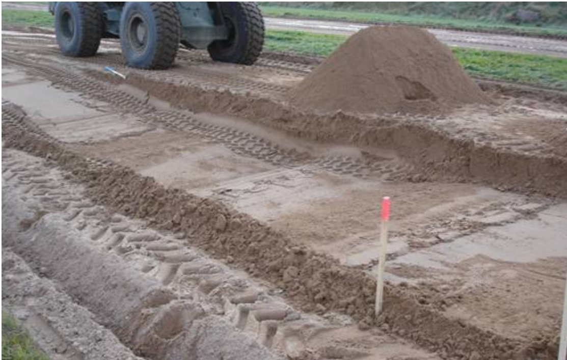
Photo of excavation from Stage 2 Phase 1 Serial 1D
