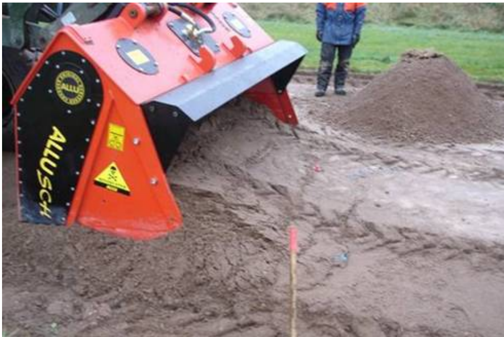
View of lane excavation nearing completion
