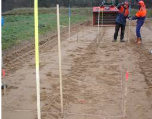
Completion of lane setup for Serial 1B Sand
