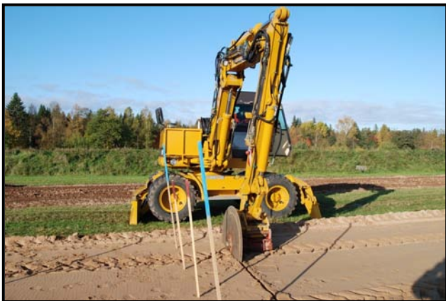
Pizza cutter being used to prepare for placement fibre boards
