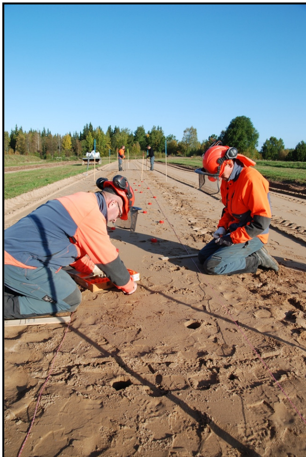
Test lane being prepared
