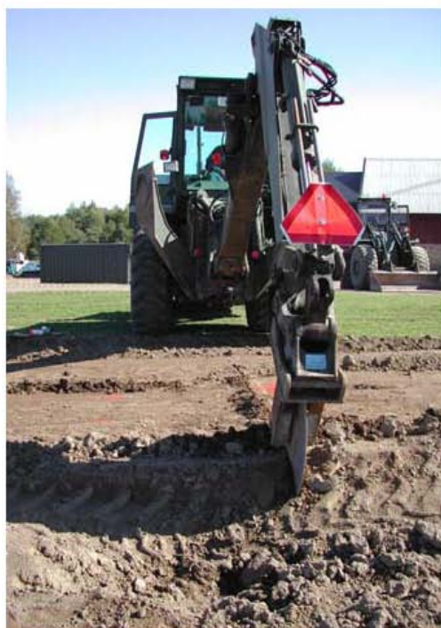
Figure A-14. 'Pizza Cutter' used to install witness panels
