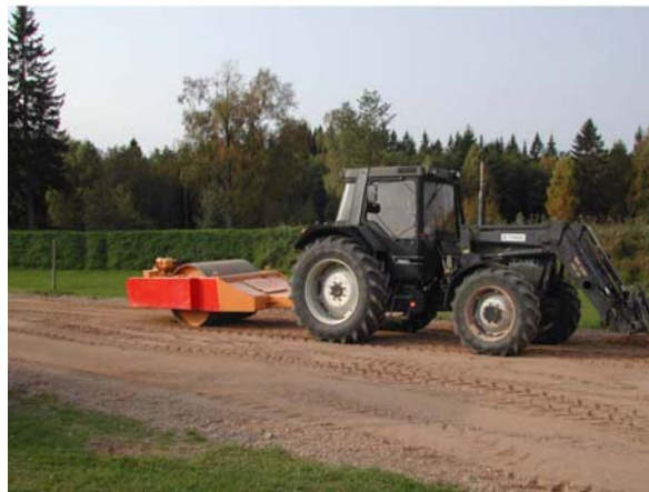
Figure A-1. Soil Preparation – Loosening and compacting the soil
