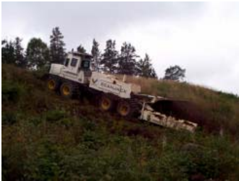
The picture shows clearing in 20% downward slope
