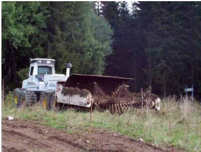
The picture shows clearing on 10% side slope
