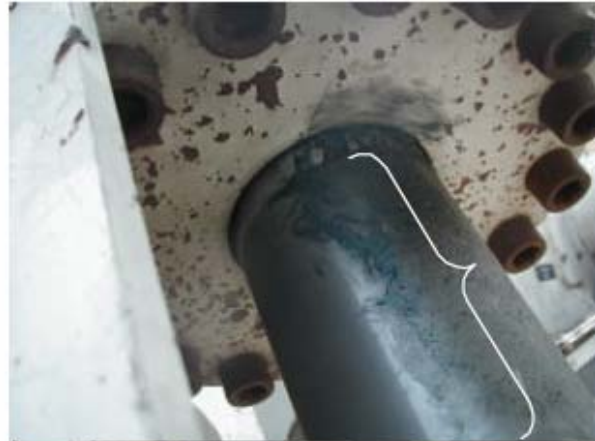
The picture shows vertical shock absorber Clamp =motion reserve
