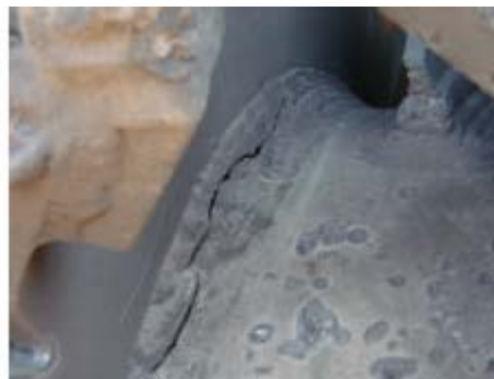
The picture shows formation of cracks in attachments of clearing arm
