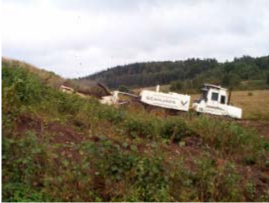
The picture shows clearing on 20% upward slope
