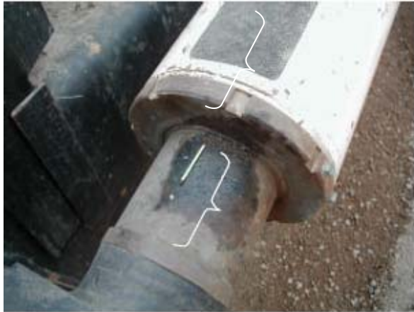
The picture shows horizontal shock absorber Clamp =motion reserve
