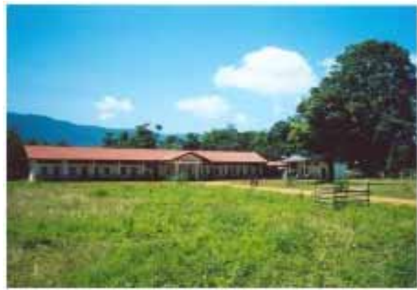
Plate 4-5 Site 2. Grounds of the Thateng Tai hospital
