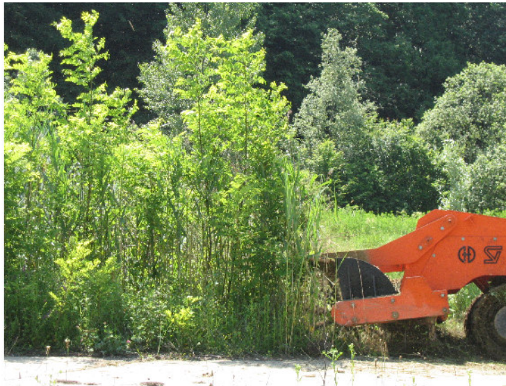
Figure 5-15: RM-KA-02 at the start of the Vegetation Clearance Test
