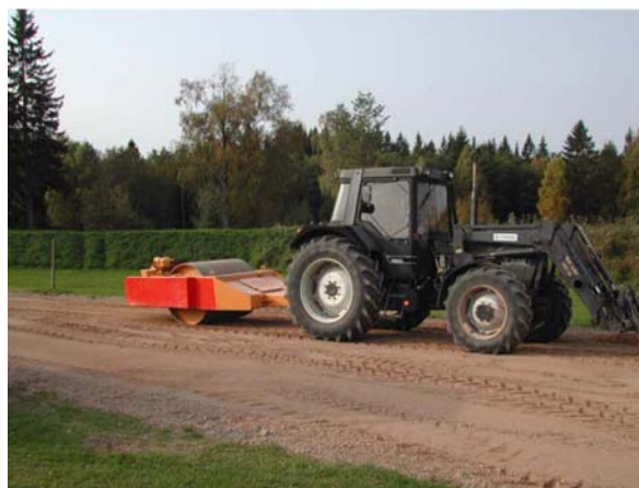
Figure A-1. Soil Preparation – Loosening and compacting the soil
