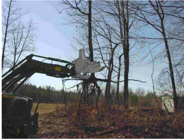
Figure 32: Tree Picker in Operation
