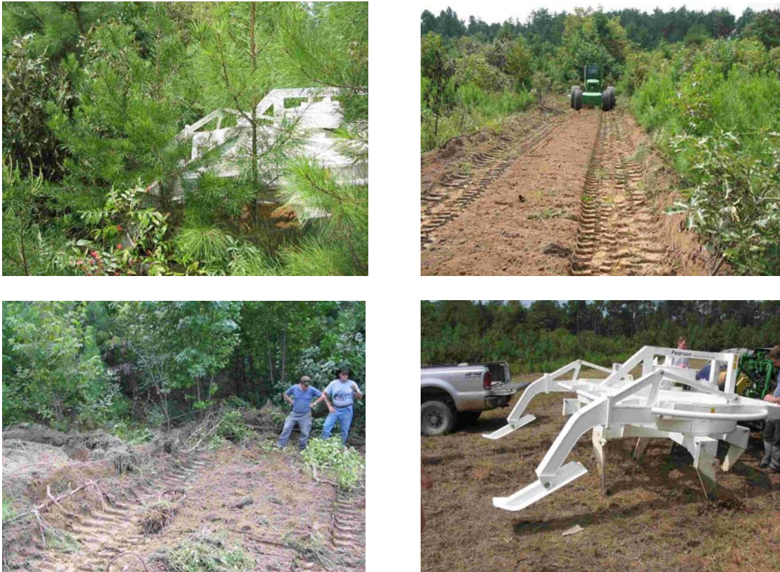
Figure 30: Rotary Mine Comb Demonstration
