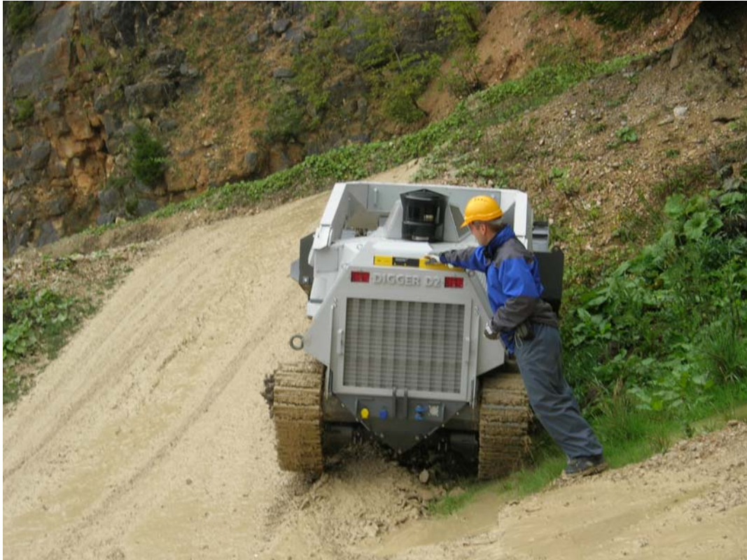
Figure 3-5 Measuring side slope
