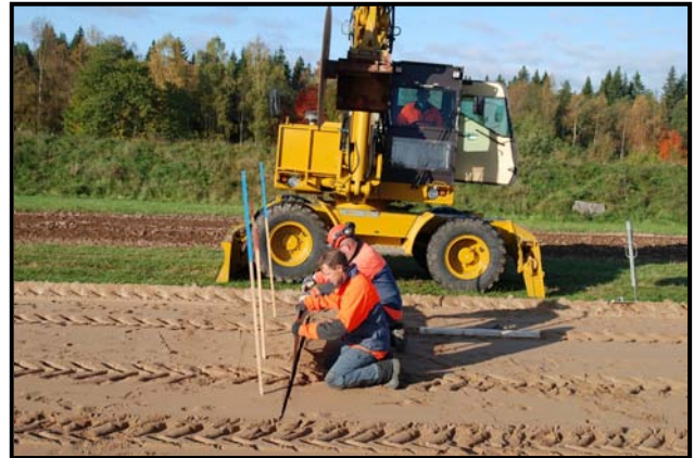
Fibre board being buried
