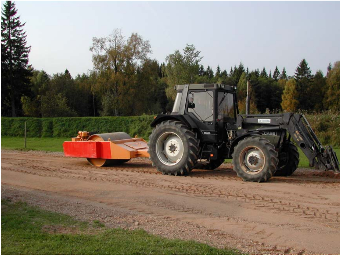
Figure 2. Soil Preparation – Compacting the Soil
